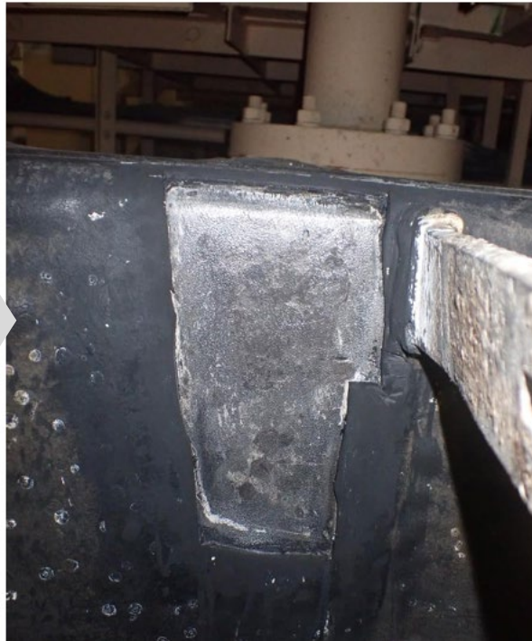
Figure: Defect Area to be repaired after removing corrosion using hand tools
