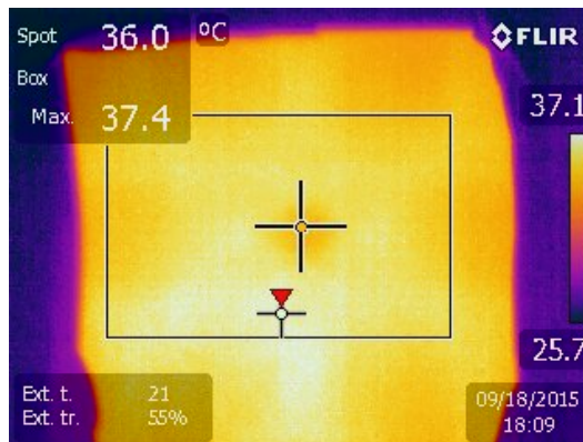
Figure 5 Thermal Image, IRISS Window Grid Lines
