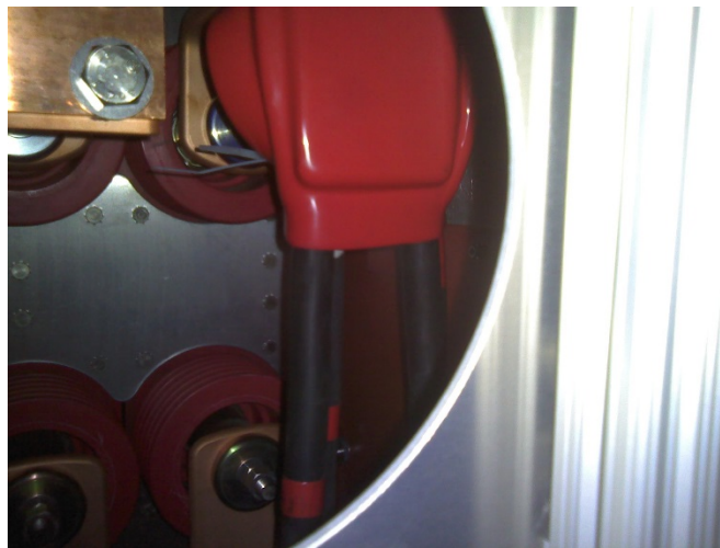
Figure 52 Visible Image, Cables below Position B, No Window
