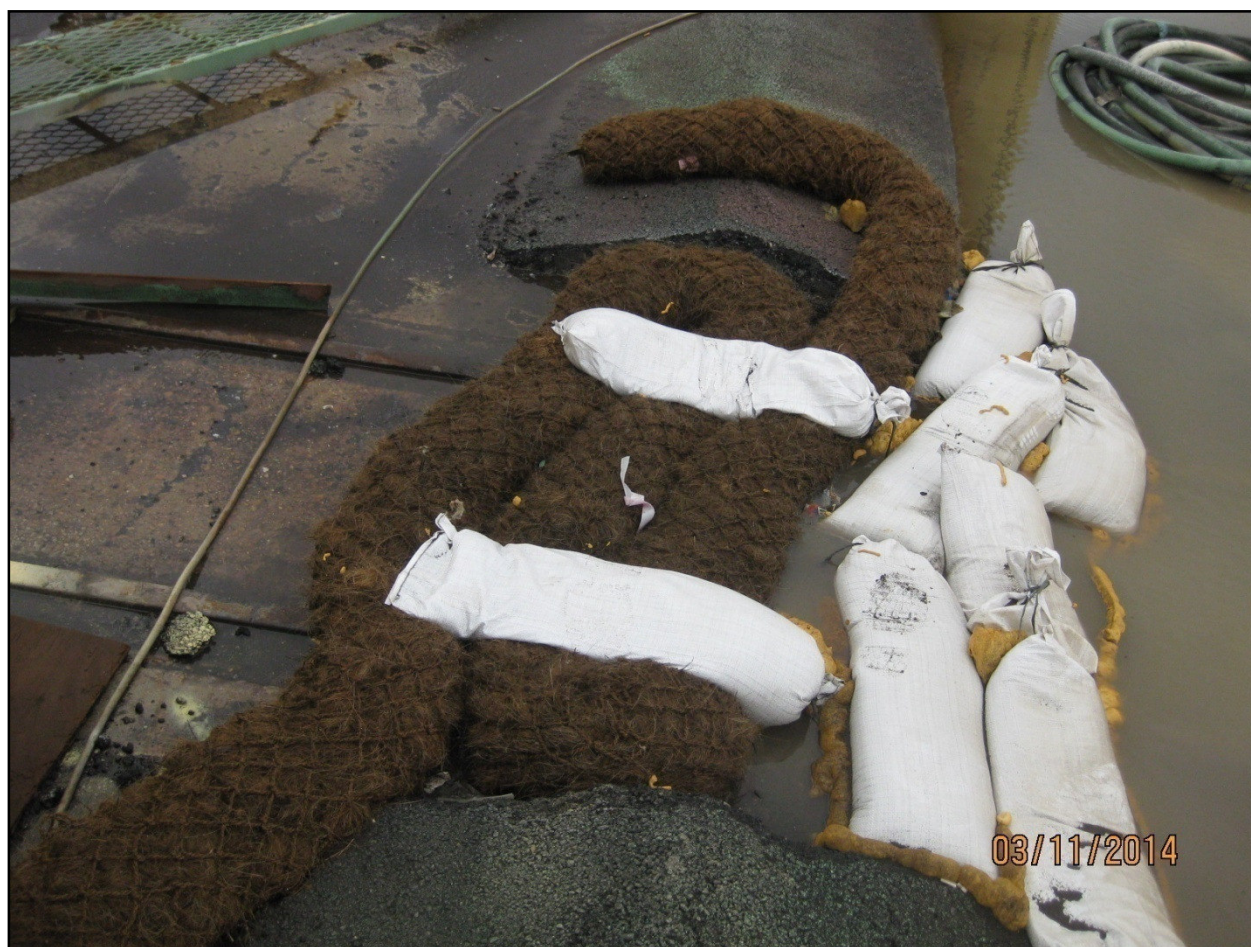
Figure 5: Slurry Pit Technology Installation
