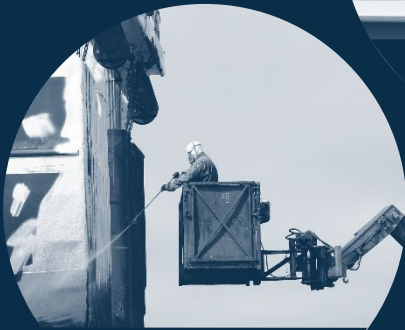
Lack of detail planning
