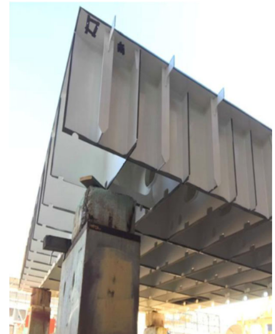
Example of MIL-PRF-23236 Type VI primed module from ship construction , Ingalls Shipbuilding, NSRP Retention of MIL-PRF-23236 Type VI Epoxy, 2019
