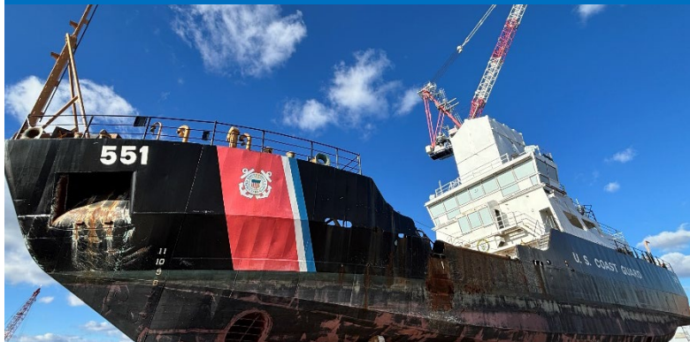
175' WLM MMA – In Progress
