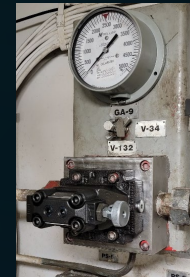
USS Wasp (LHD-1) Aircraft Elevator High Pressure Air Reducing Manifold
