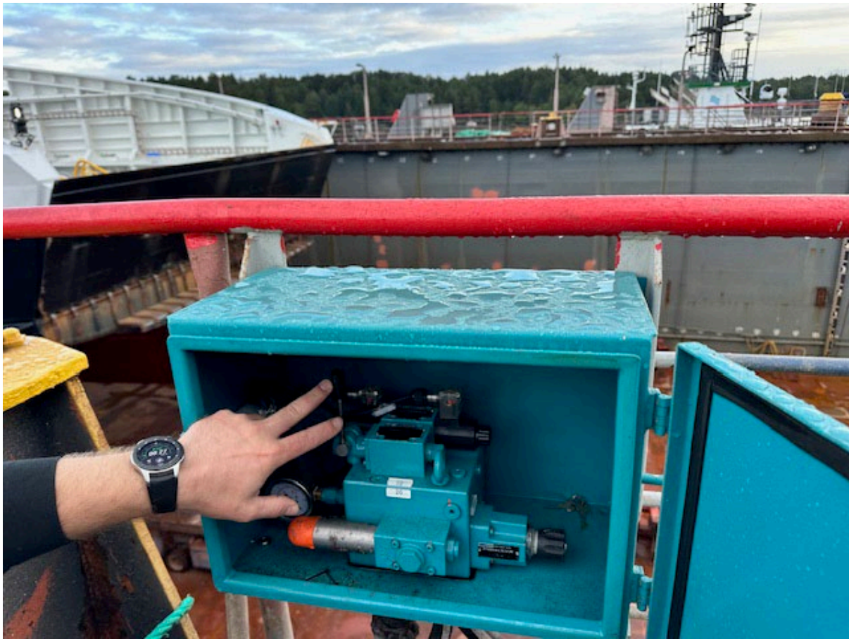
Figure 6: Photo of Bilge Support Arms Local Controls
