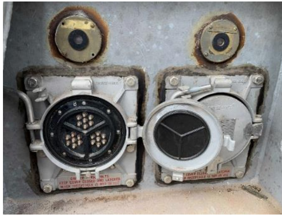
Figure 16: Shore Power Receiving Station (Two of twelve receptacles shown)
