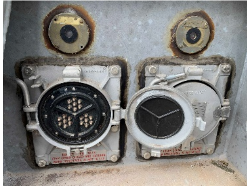
Figure 13 Two starboard most receptacles with indicator lights above
