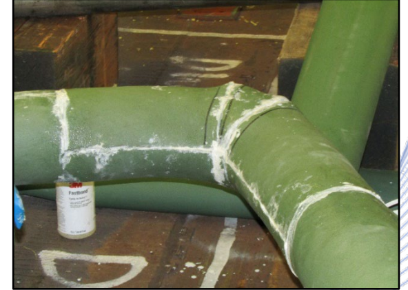
Gluing pipe seams
