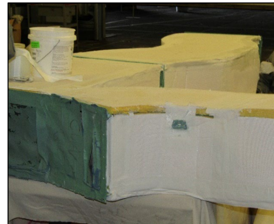
Vent duct fitting, gluing, and taping
