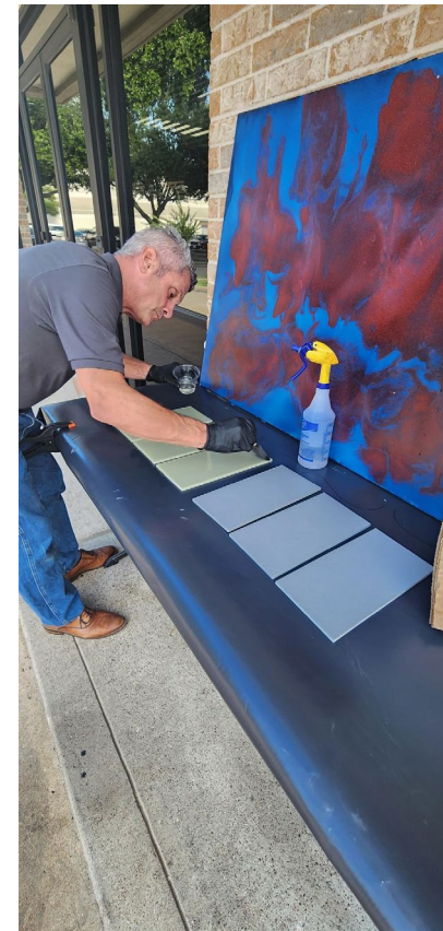
Application of coating to panels at Coval Technologies provided by Jason Dixon
