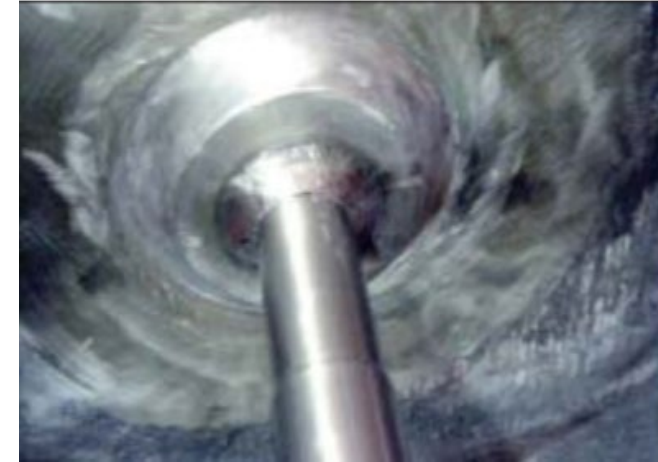
Ambient Temperature Temper Bead Weld Metal Buildup for Alloy 690 Instrument Nozzle Repair
