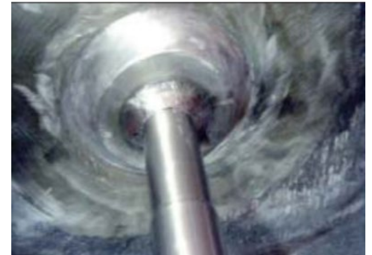
Reactor Vessel Instrument Nozzle Repair
