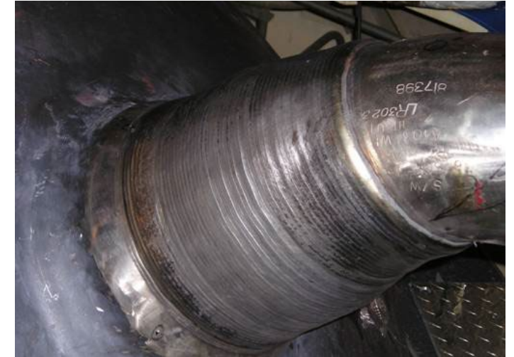
Pressurizer Relief Nozzle Weld Overlay
