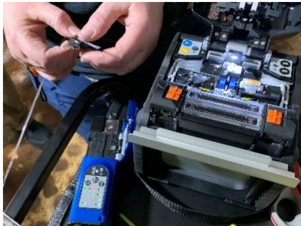
Figure 15. Installation of Ribbon Fiber in Holder
