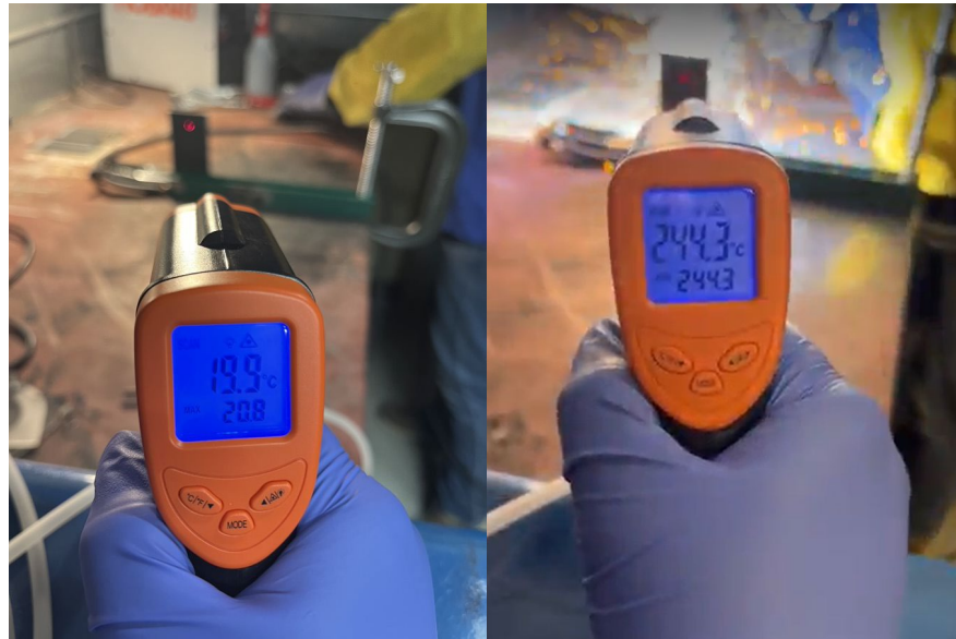
Before Welding 19.9C (67.8F)
