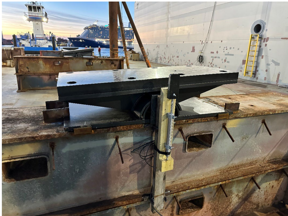
Figure 13: Docking 3 HDPE Side Block Before Docking
