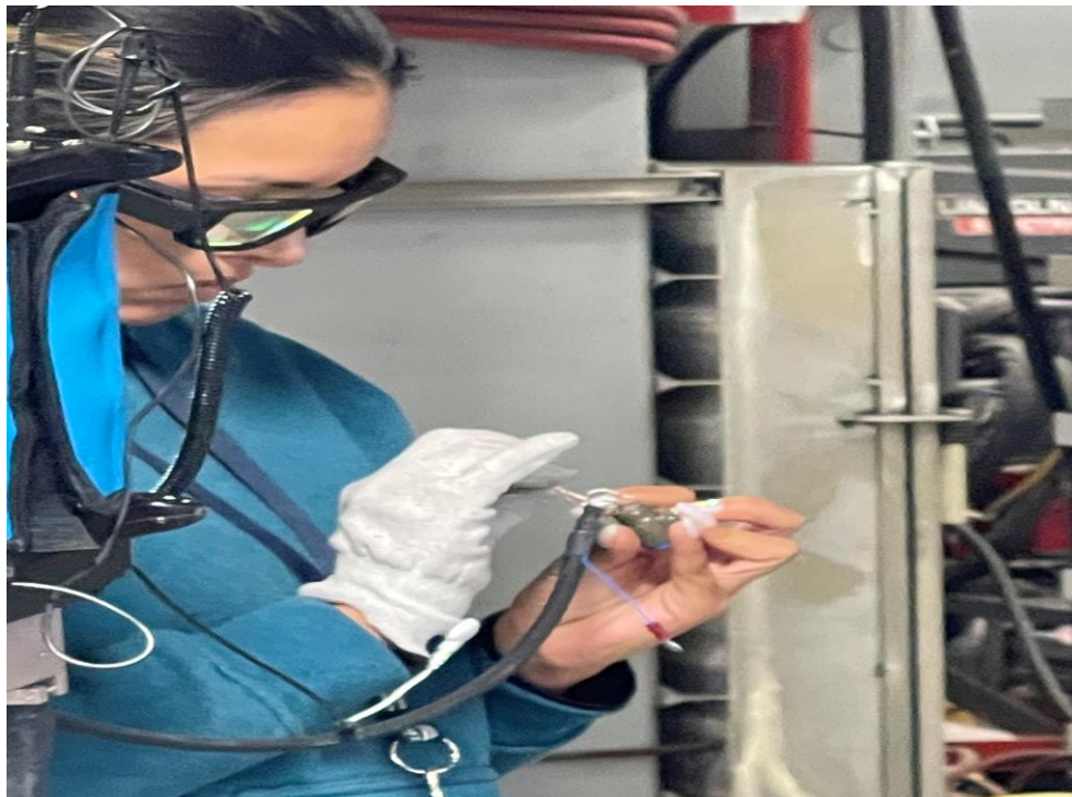
Figure 11. AMUET 4.0 assists production, it allows a shipboard electrician to use a smart lens to prepare and perform the conductor insertion at the cable's connectors, using AMUET proprietary patented processes. This allows the technician to use both hands and reduces fatigue by avoiding repetitive readouts of wire numbers/colors from manuscript documents. No programming is required to use this feature. Lussier US patents 9817942 and 10705135.
