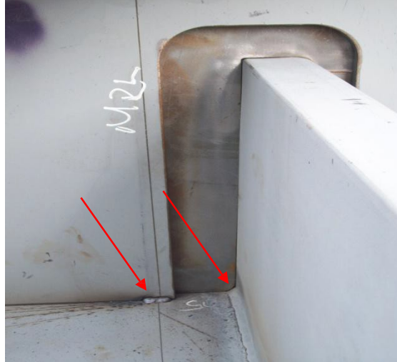
Figure 27 – Tack welds
