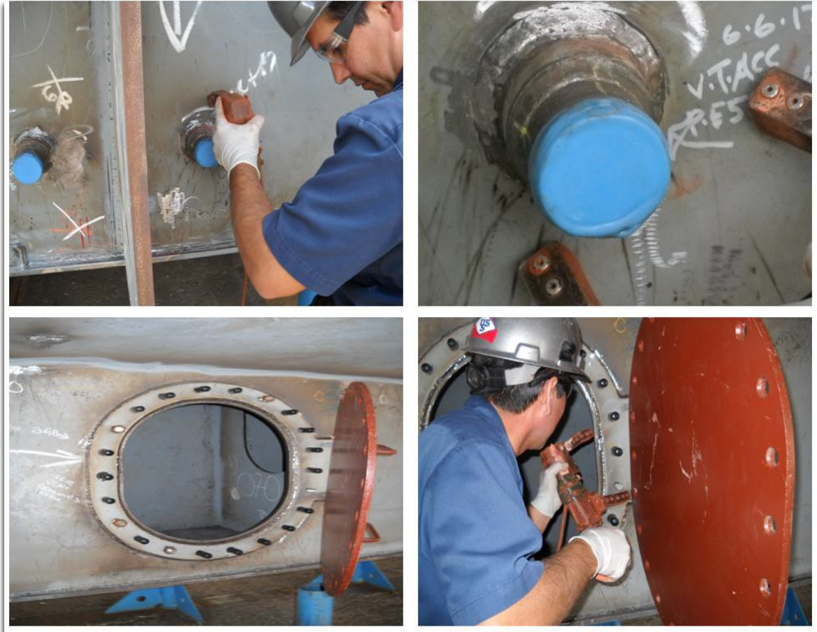
Figure 5b – Tank pipe and manhole penetrations being tested
