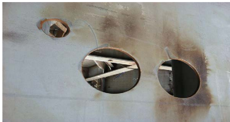
Figure 22 - Multiple penetrations through tank boundaries
