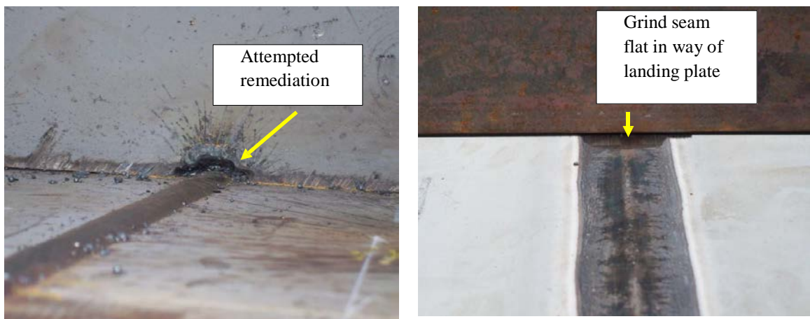
Figure 16 – Parts crossing weld seams
