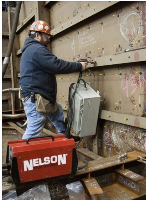
Figure 15. Pinning at BIW with N800i and energy monitor
