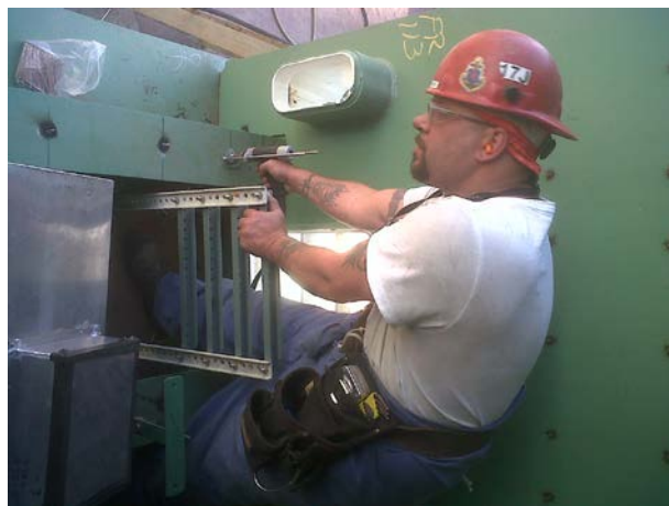
Figure 9. Insulation pinning at Ingalls
