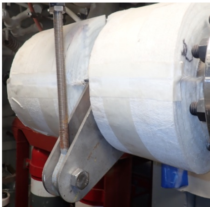
Insulation Tape Before Lagging
