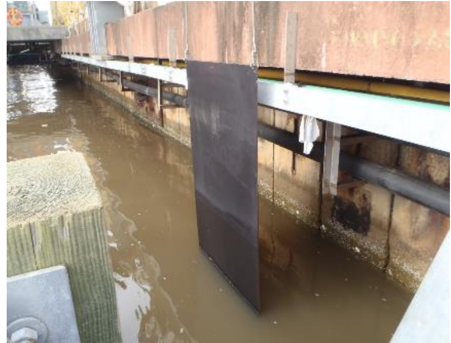
Panels submerged at HII in January 2020
