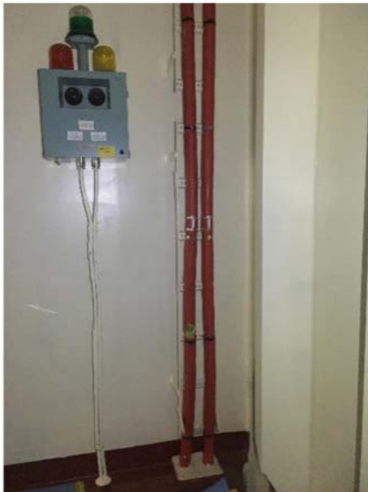
PC76 : Install Cable Protection
