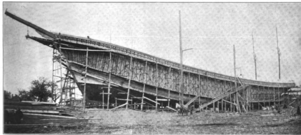
THE LARGEST WOODEN SAILING VESSEL EVER BUILT. NOTE THE DIAGONAL BRACING OF THE HULL.
