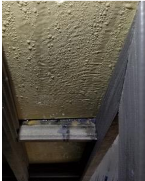
Figure 14. Panel in Condensing Test
