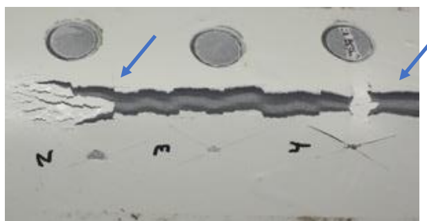
Figure 18. Damaged areas displayed less delamination.
