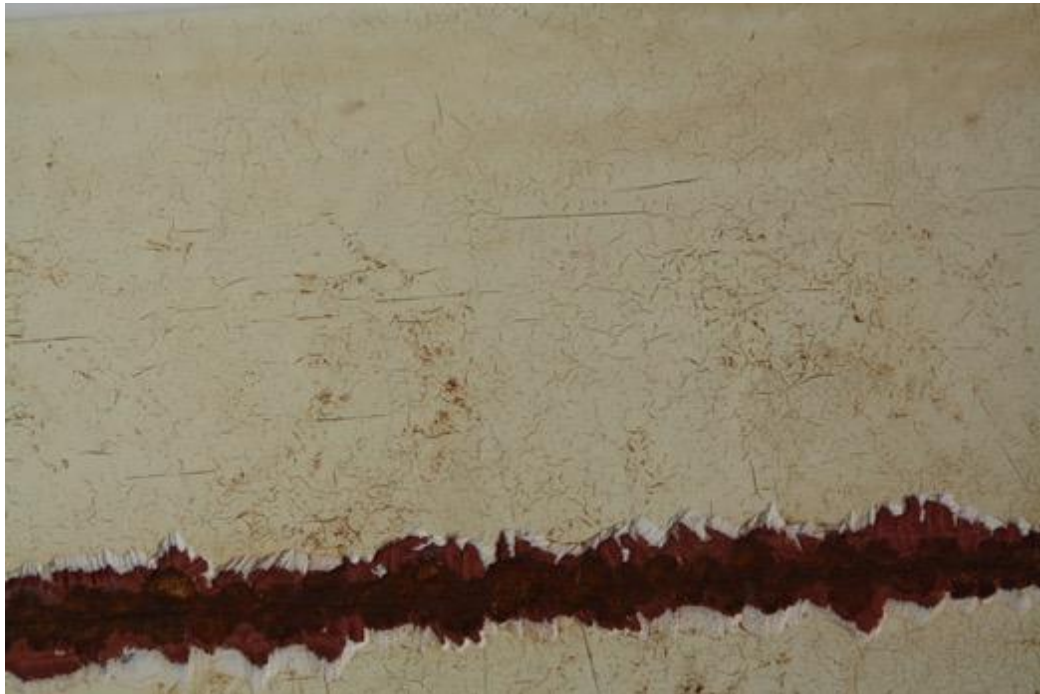
Figure 24. Checking on Interbond 998 Topcoat
