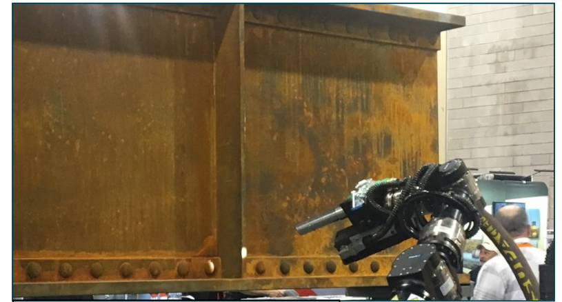
Robotically abrasive blasting a beam: Elzly photo
