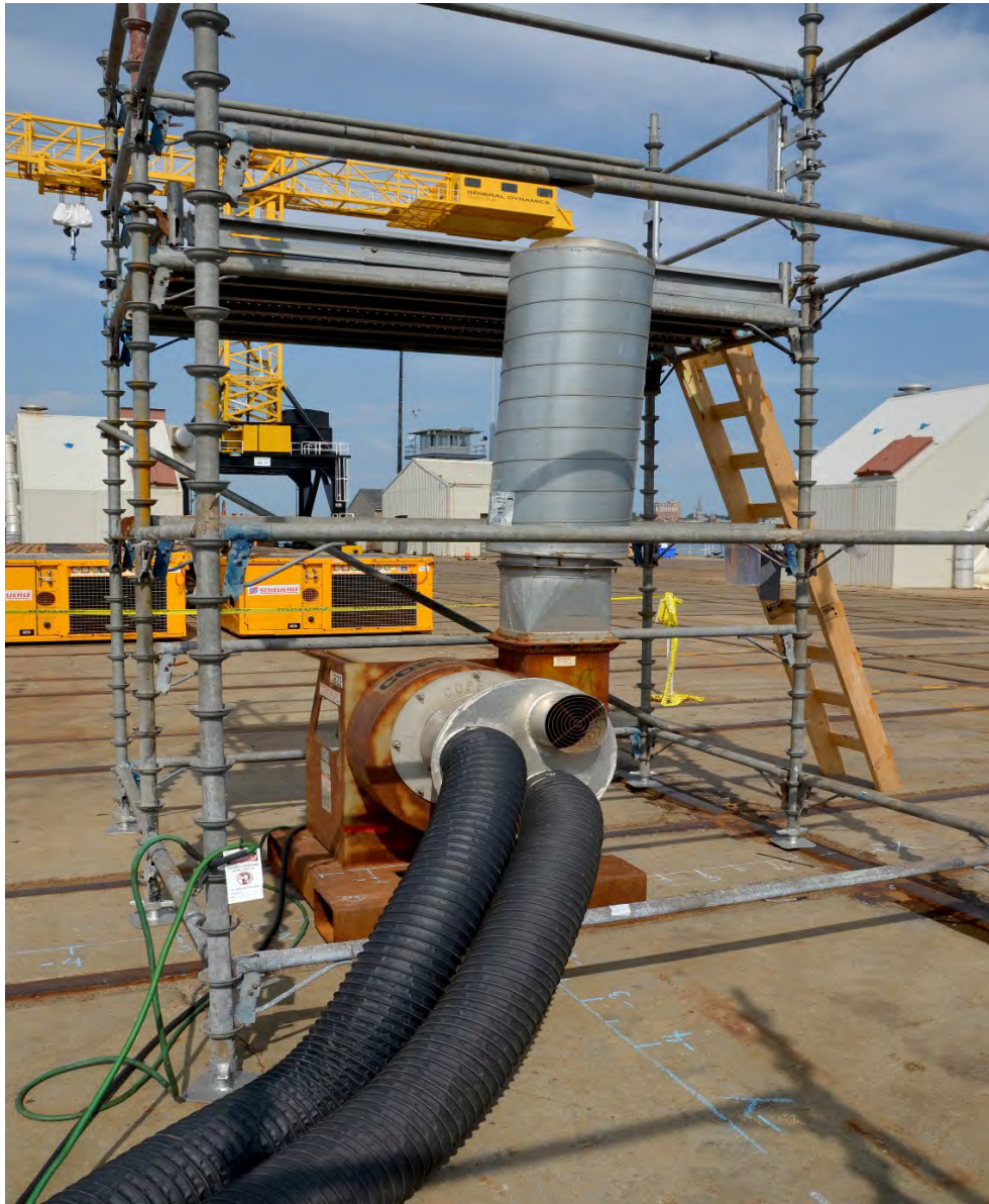
Figure 8 – Coppus TM-8 Test Area
