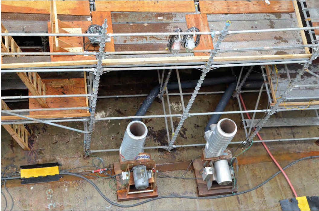
Top View, PVB Units in Drydock
