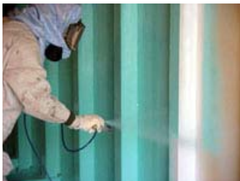
Figure 3 – Protective Equipment for Shipyard Painting (Source: OSHA Shipyard Employment e Tool – Painting and Other Coatings)
