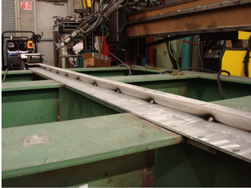
Figure 6.5: Tacked Stiffener Test Assembly on Test Frame
