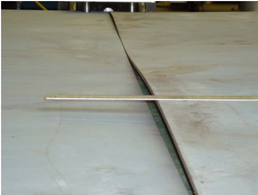
Figure 4.7: Fit-Up of Plates before Pre-Tensioning
