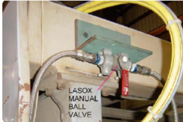
Figure 35: Manual operated ball valve LASOX oxygen gas control assembly
