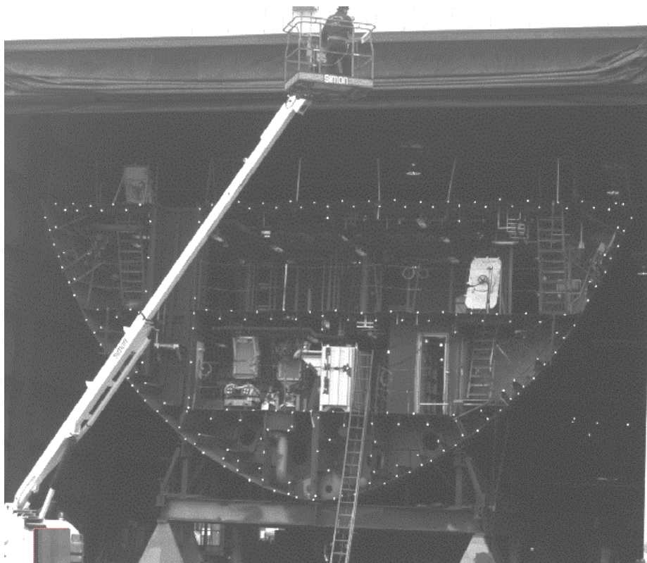
Figure 5a – Unit end measurements to determine unit make-up alignment accuracy
