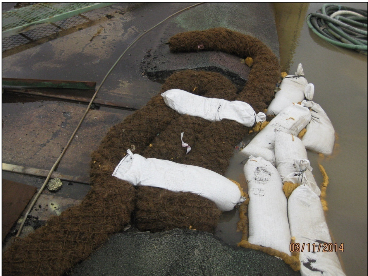
Figure 5: Slurry Pit Technology Installation
