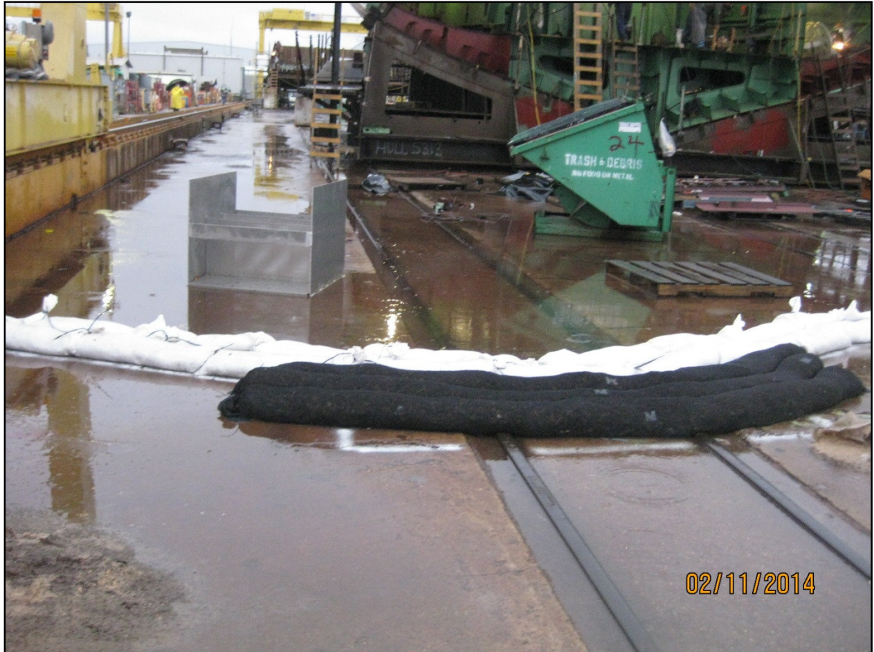
Figure 3: Control technology installation at production bays.
