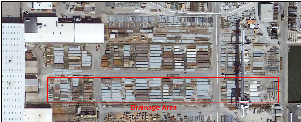
Figure 1. Aerial of Plate Laydown Yard
