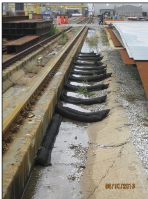
Figure 12. View of Plate Laydown Yard During Discharge Event
