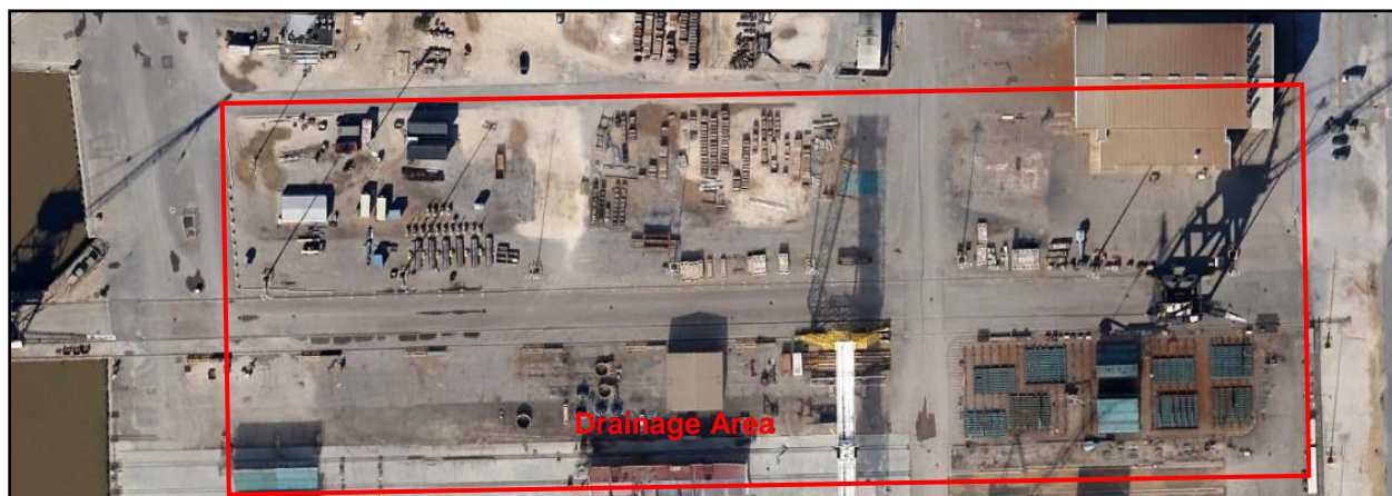
Figure 4. Aerial of Crane Track
