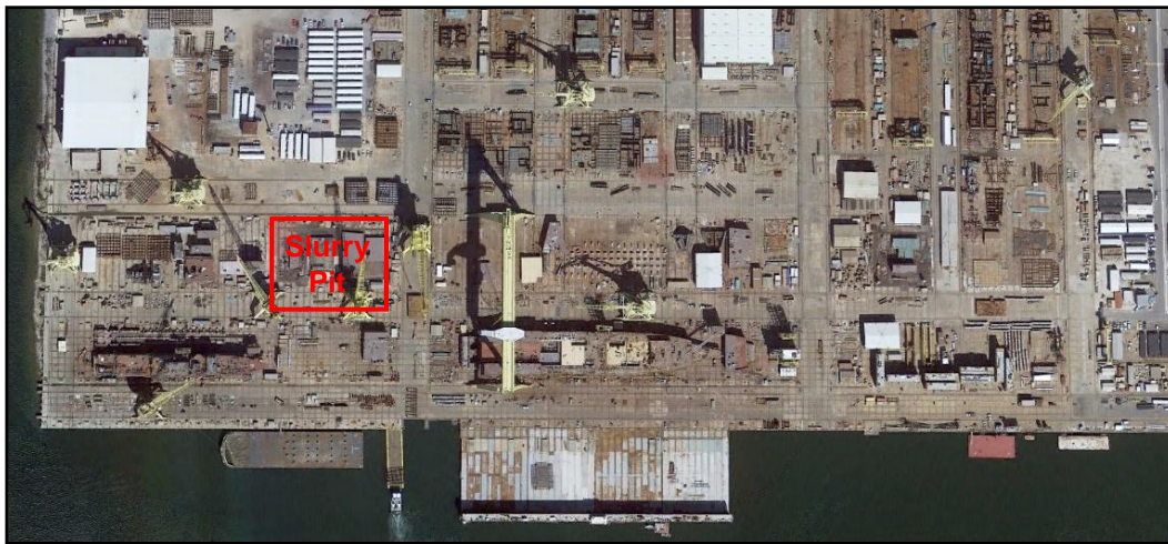
Figure 2. Aerial of Slurry Pit
