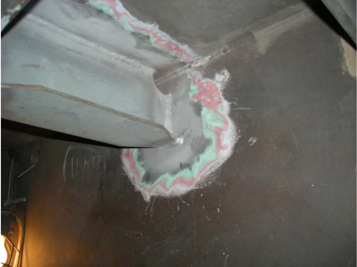
Figure 3. Installed stiffener with PCP surface and welds prepared for painting.
