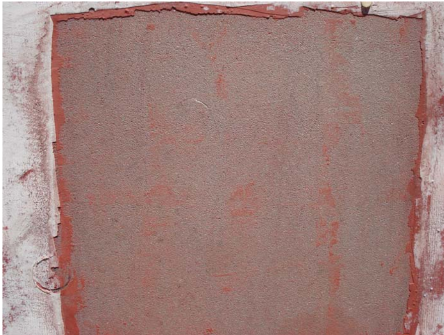
Figure 9. Test patch 4 with nominally 100 square inches of coating removed.
