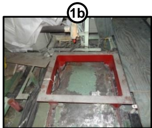
Rig Foundation into Place, Protect Adjacent Areas for Welding Operations, and Tack Foundation in Place
