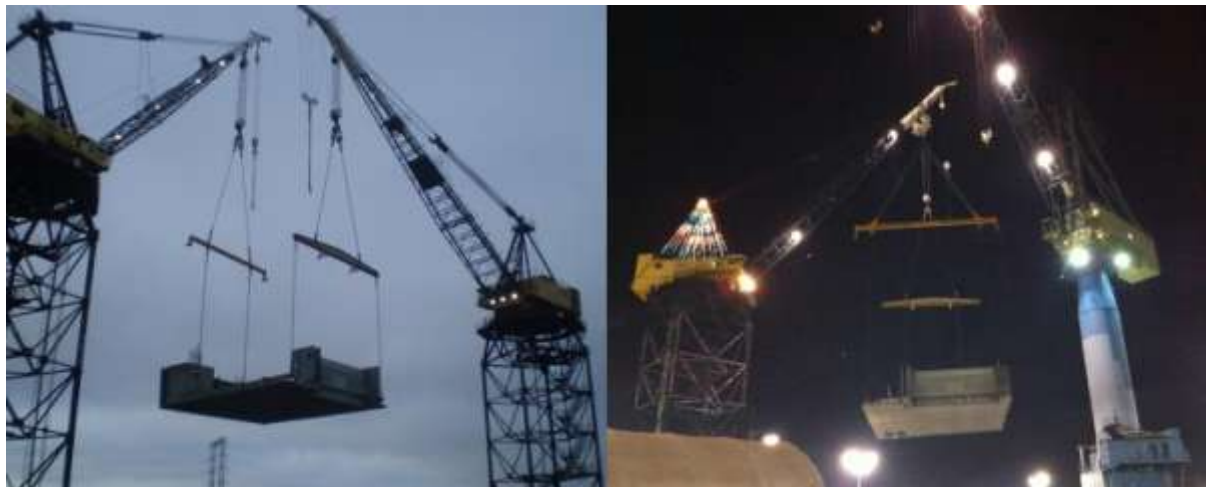
Figure 7: June 7, and Dec 8, 2010 Deck and Shell Block Lifts
