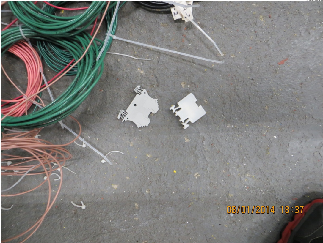
Photo 21 – File No. AG14-1052 View after Shock Blow No. 3 in the back direction, parts flew off and came loose
