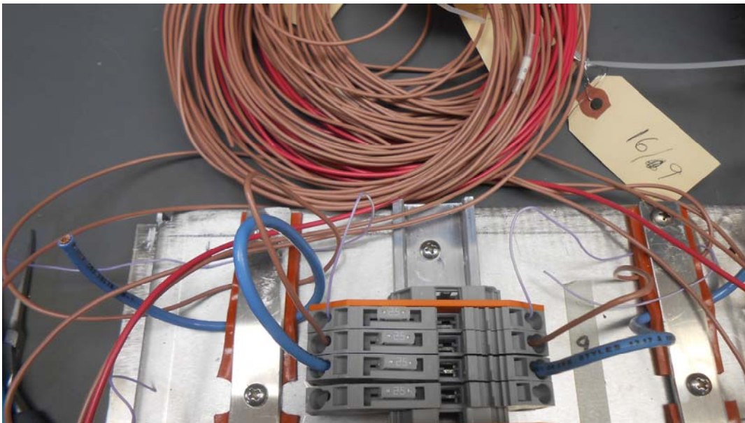
Figure 5.5-36 Conductors Coiled for Instrumenting Test Article
