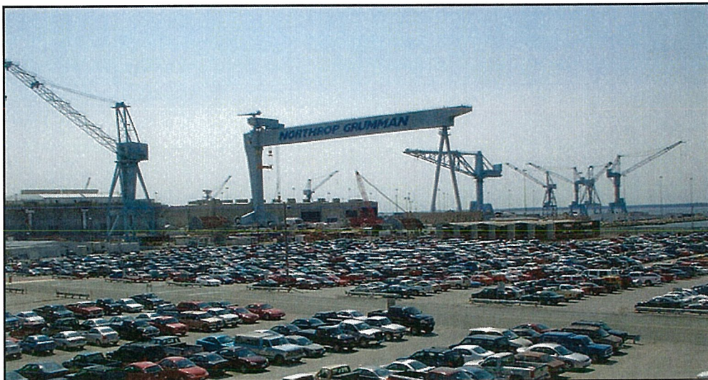
Figure 1 – NGSB 1050 Ton Gantry Crane
