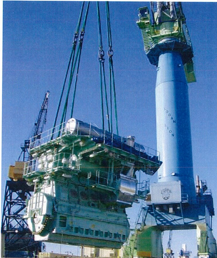
Figure 4: Lift Operation for a Ship Engine
