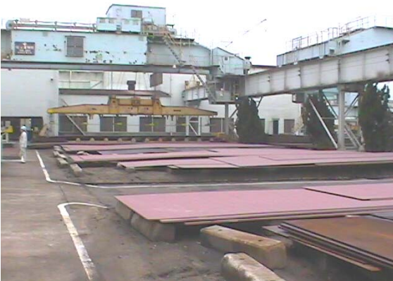
Photo 28: Frequent Delivery of Steel Minimizes Inventory
