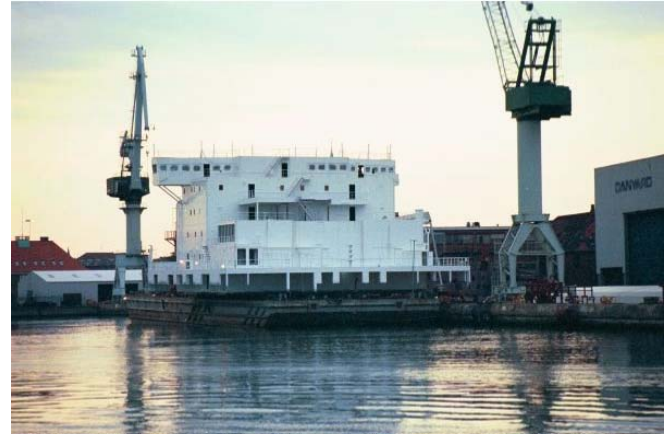
Photo 31: Turn-key Sub-contractor Deck House
