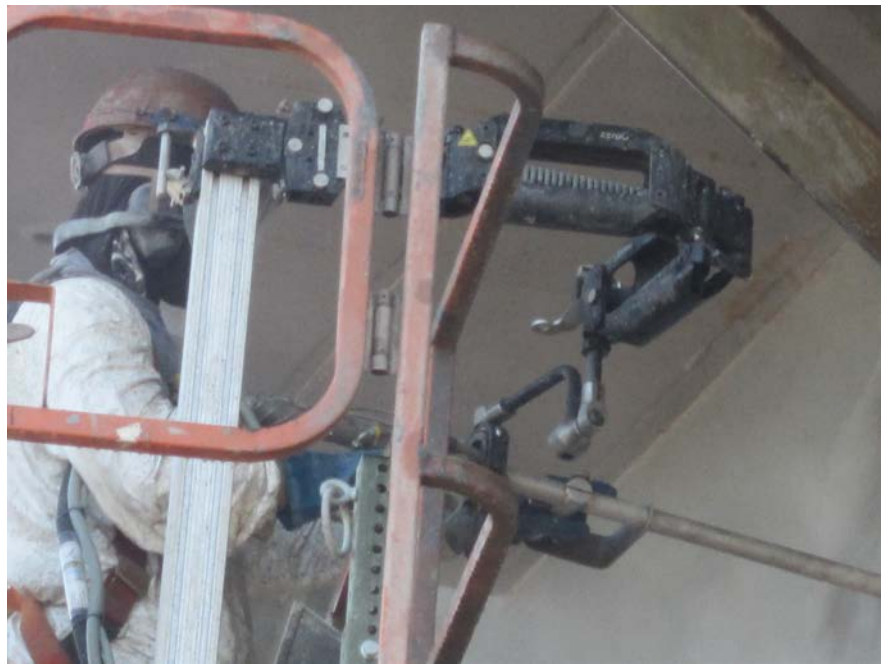
Figure 3. Water Jet Lance on Man Lift
