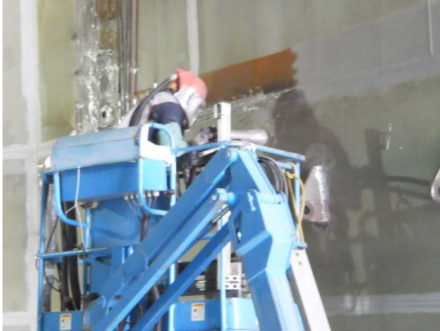
Figure 6. Abrasive blasting using zeroG System
