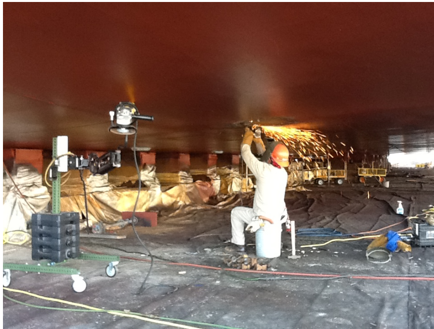
Figure 4. Overhead Grinding without zeroG Arm
