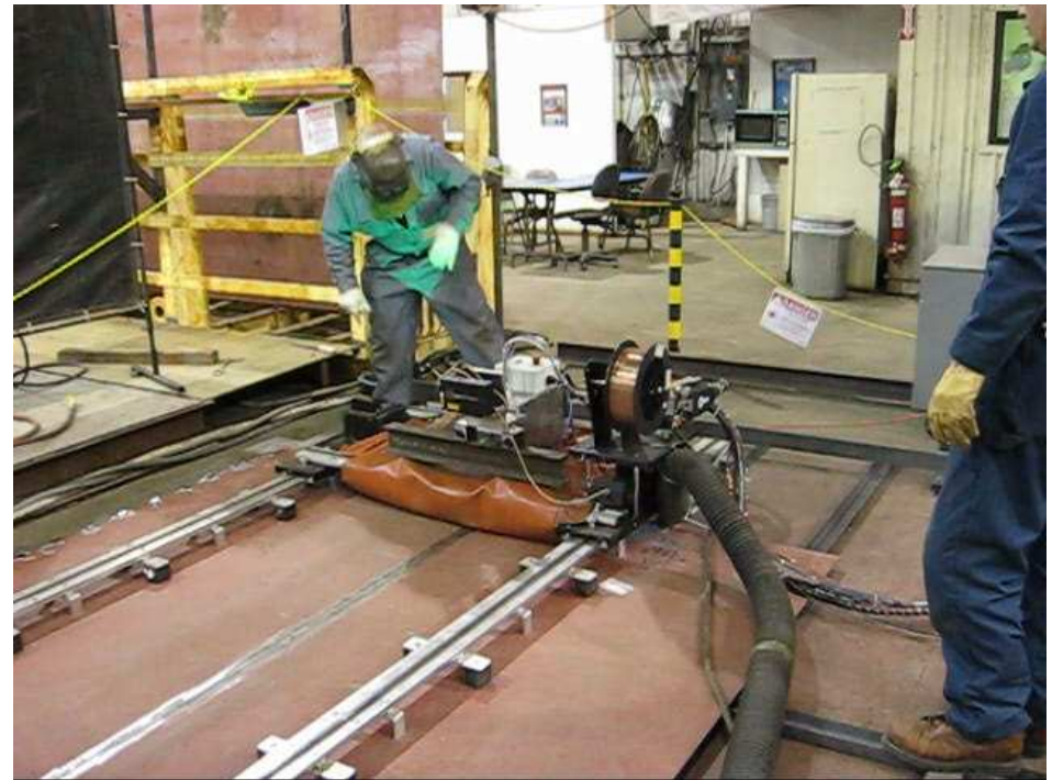
10ft panel HLAW weld at BIW on 17 Jan 2008
