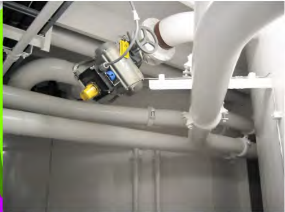
Picture of the actual bulk mud fill and discharge lines.
