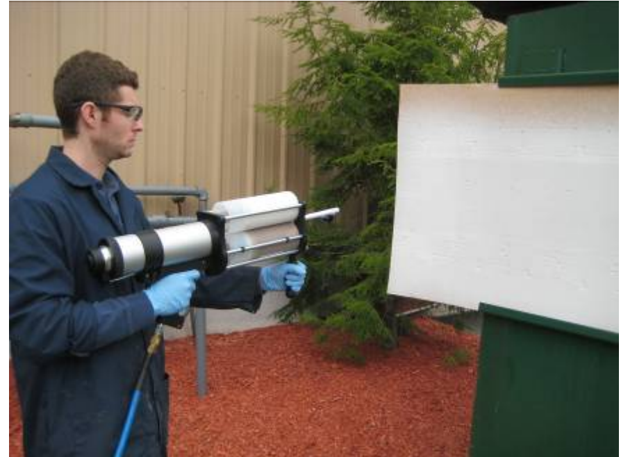
Application with the cartridge spray system
