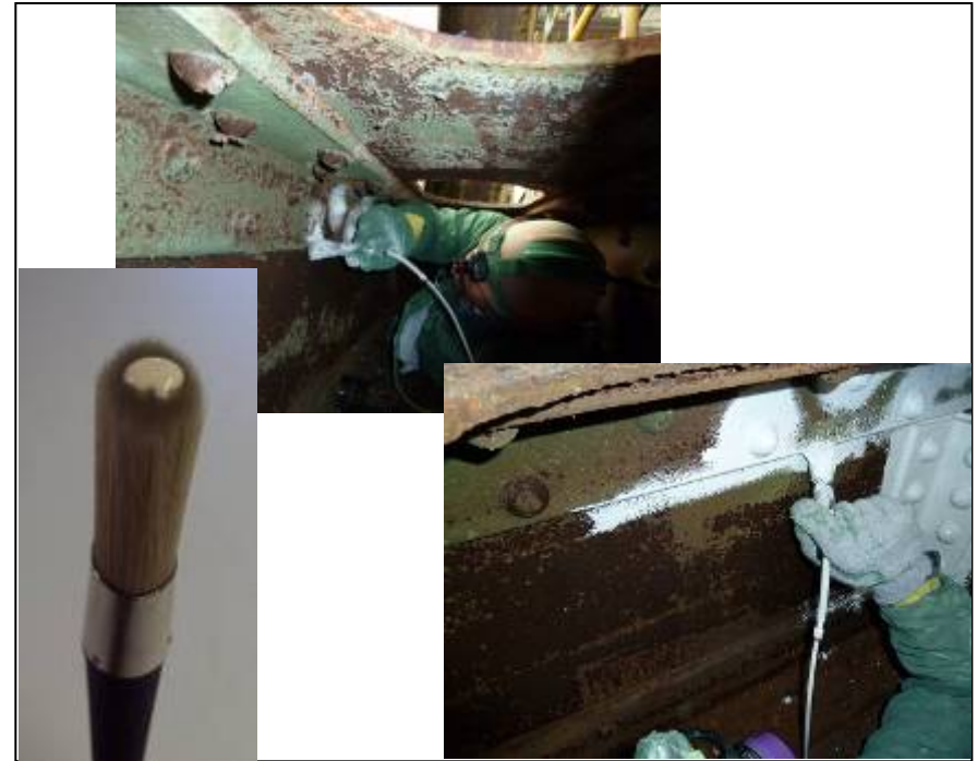
Application with the new flex hose brush system
