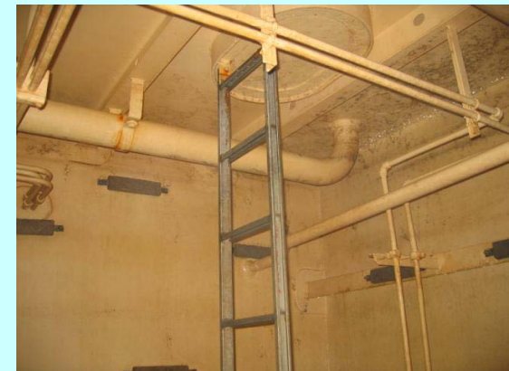
Ballast Tank after one year.
