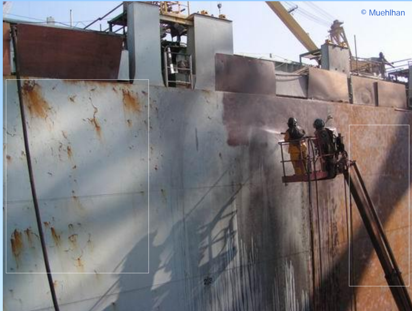
Rust degree on coated surfaces (ISO 4628-3)
