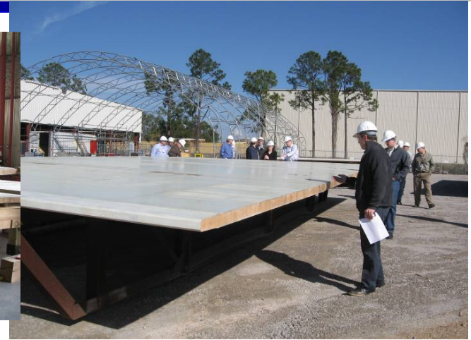
20' x 40' Assembled Test Panel
