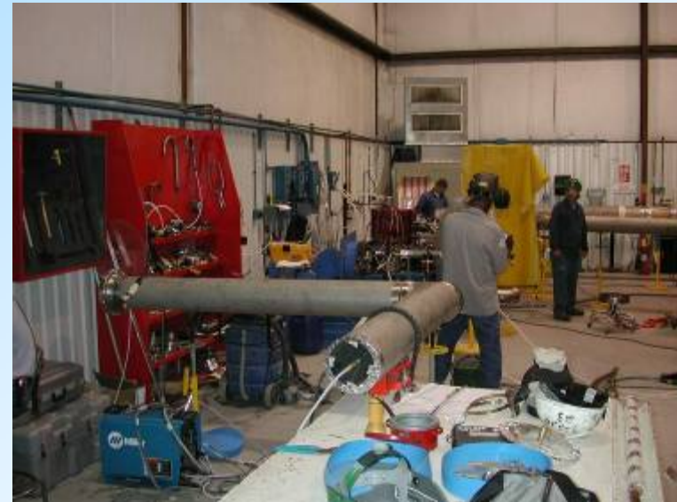
NGSS Avondale Titanium Fabrication Facility for Piping Subassemblies
