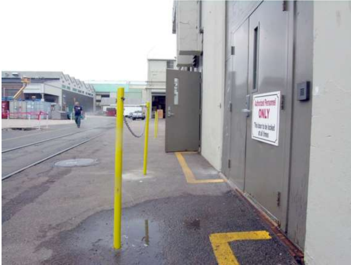
Posts protecting doorways into roadways.
