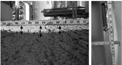
Ship Superstructure Plate Deflection Between Structural Members
