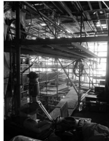
Structural Ship Alteration Expanded for the Gas Turbine Air Intake on Specific CG-47 Ships to Renew Adjacent Aluminum Alloy Plate
