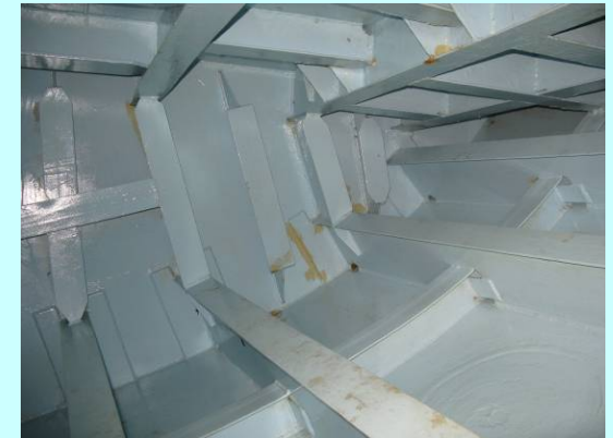
July 2009, areas touched-up using paint cartridges showing color difference. Minor corrosion at rat-holes
