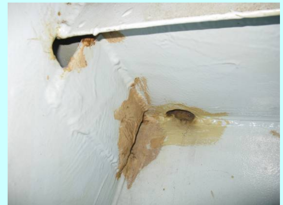
July 2009, areas touched-up using paint cartridges showing color difference. Minor corrosion at rat-holes
