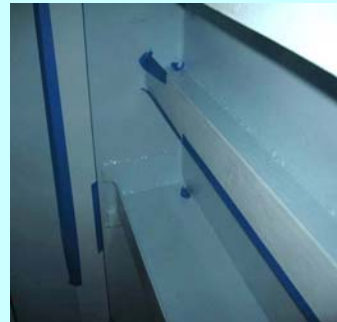
Blue, extended release masking tape indicating areas requiring paint touch-up. Final job accepted by QA
