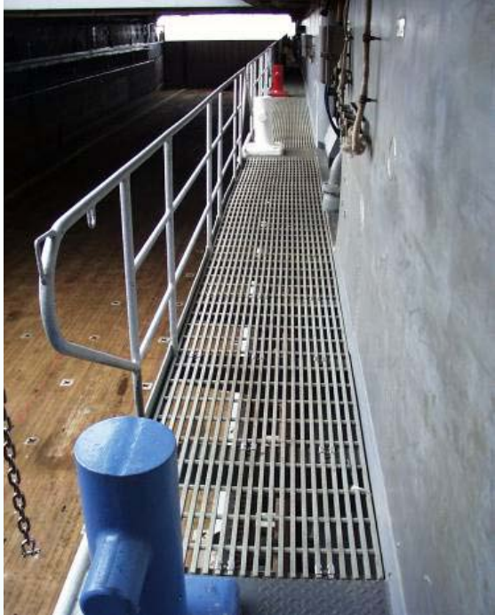
LSD Wing Wall
